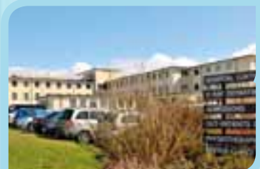
Merlin Park University Hospital
